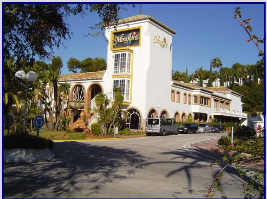
Centro Miraflores South & East Facade
